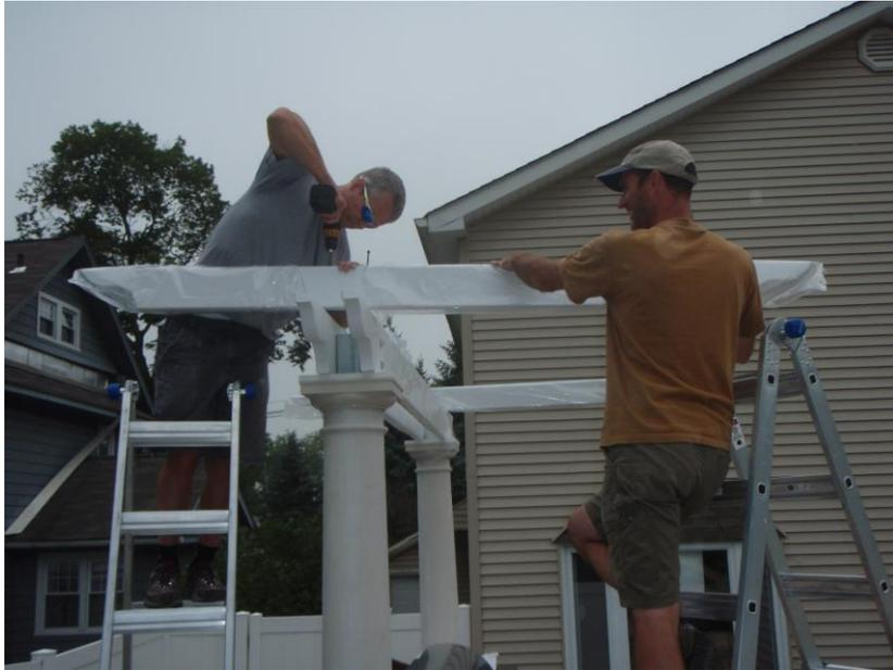
Leave protective plastic on the rafters when installing to help keep rafters clean of handprints. Set back screw first, check level and set front screw. Be careful not to overtighten.
