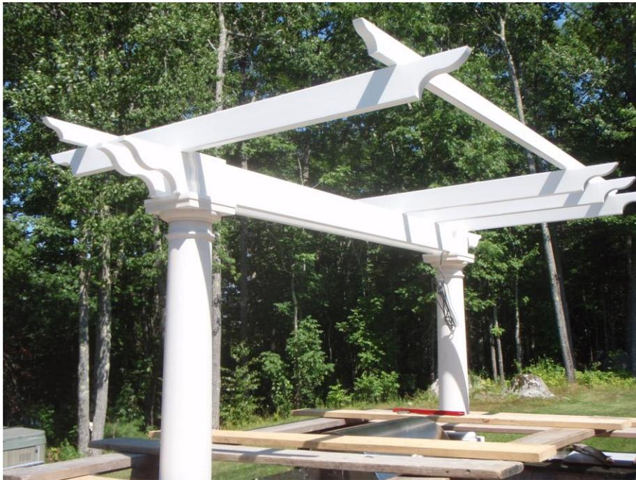
Set then and level the leftmost and rightmost rafters first. Then set the backmost and frontmost purlin. Double check level on both rafters and purlins. Begin installing the remaining rafters and then install the remaining purlins.
